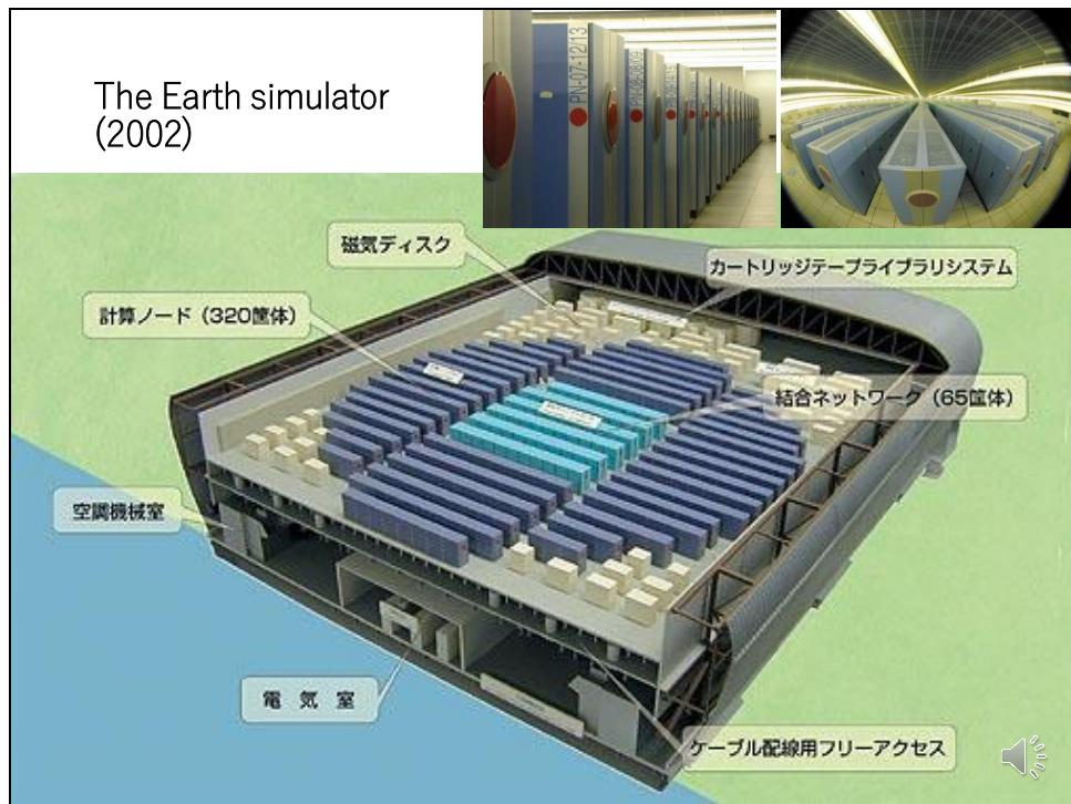
The Earth Simulator got the top 1 in the world 2002. A lot of cabinets are placed on the big building like a gym. The deep blue ones are for computational nodes and light blue ones are for interconnection networks.
